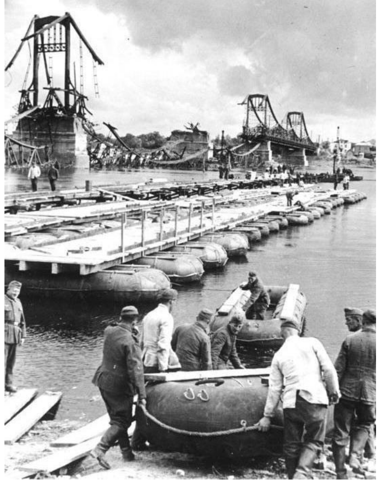
During the First Battle of Kiev, this pontoon bridge over the Dniepr was constructed in a day. The Germans encircled Kiev, which fell to them September 26, 1941 after three months of siege. Of the 400,000 plus soldiers in the city only 15,000 escaped. In retaliation, the Soviets conducted a scorched earth policy that included destroying as much of the city as possible.
