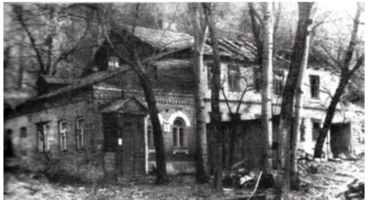
Building also numbered #5-B Vozdvizhenskaya Street. Kovalinsky thought it might have belonged to someone in the family but that is uncertain. Still, it certainly belonged to neighbors they knew. The building is in a different style from the typical Podol houses but the address is correct as it was carefully labelled. (Photo Credit: Oldkiev.top).
